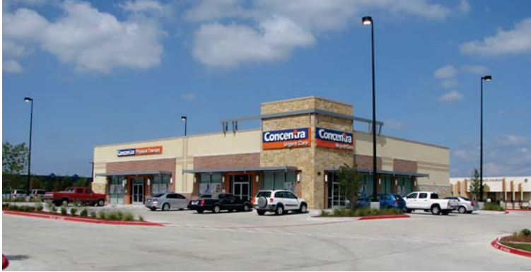
CONCENTRA AT HIGHLANDS EAST
