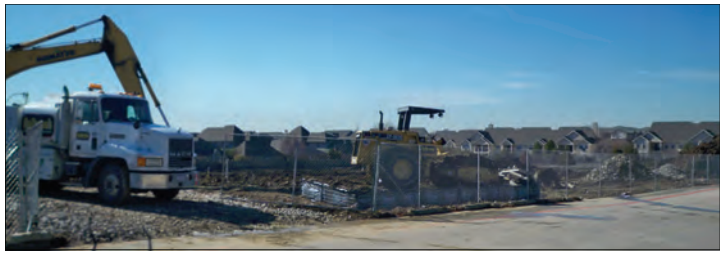
LEGACY AT BEAR CREEK CURRENT CONSTRUCTION
